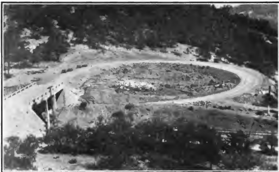
PACIFIC HIGHWAY DESCRIBES A LOOP IN WHICH IT CROSSES ITSELF AND A DOUBLE TRACK RAILROAD. Elevation, 4,500 feet; location, north slope of Siskiyou Mountains.
